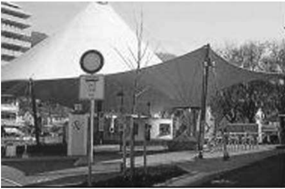
18.25 Railway and bus stations architectural membranes [65].
